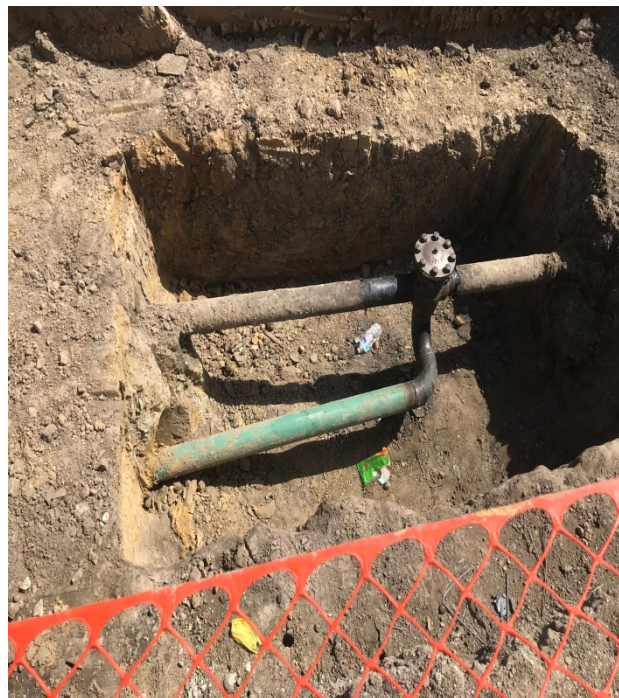
CenterPoint Gas relocated line
