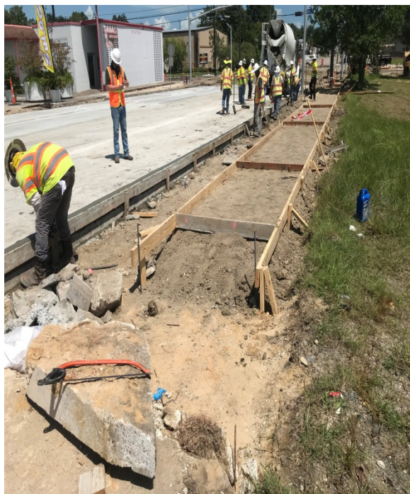
Sidewalk forming work at W. Texas Avenue
